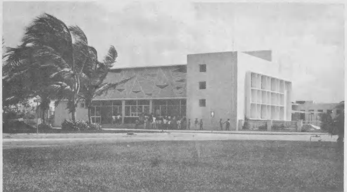
After 1-1/2 year reconstruction, an airconditioned Cultural Center was reopened June 21. The modernization had cost Fls. 480,000, bringing the total cost to over Fls. 900,000. Despues di 1 1/2 anja di reconstruccion, un Centro Cultural aireacondioná a ser re-inaugurá Juni 21. E modernization di Fls. 480,000, a trece e costo total na mas di Fls. 900,000.
